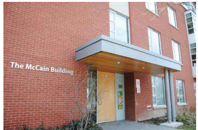
Transitional housing for CAMH’s geriatric patients is located at the McCain Building on White Squirrel Way at the Queen Street site.
